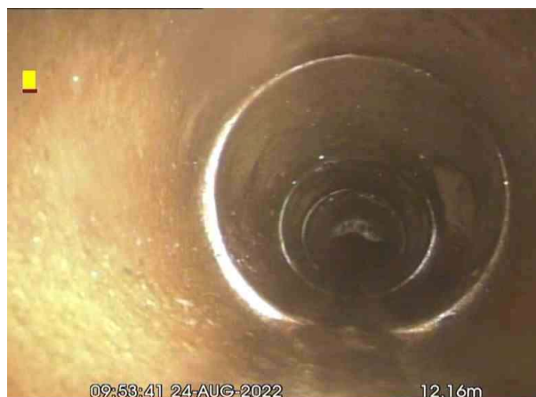
FMH4X_d52bada0-9063-49a8-9b20-ceb42b8be696_20220826_141905_096.jpg, 00:00:40, 12.16 m Line deviates right
