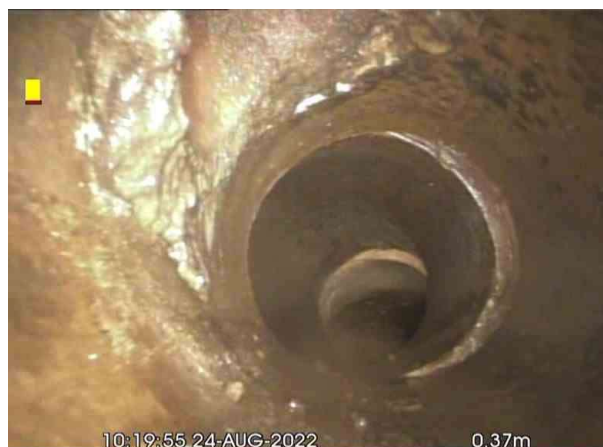
FMH7X_22c38e2c-a497-49a9-80a5-db67249a7b87_20220831_111515_842.jpg, 00:00:08, 0.37 m Connection other than junction at 10 o'clock, 100mm dia
