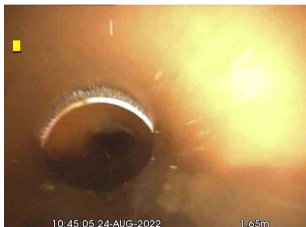
AX_b86a5d62-cf0d-4d0b-b385-77dd92a516f6_20220830_121 949_040.jpg, 00:00:13, 1.65 m Joint displaced, medium
