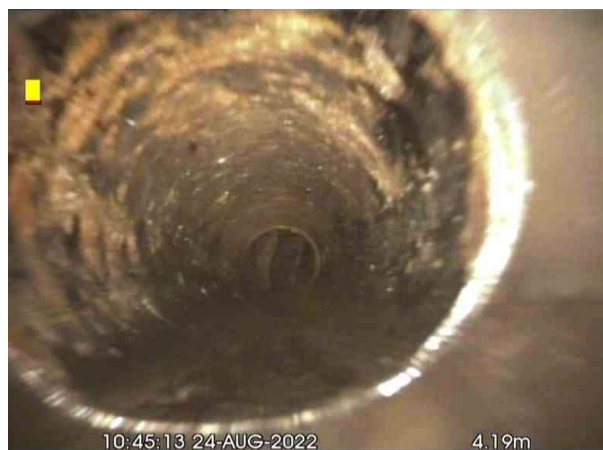
AX_7ebb41a0-5632-461a-ae39-fd359fe7652f_20220830_122 143_174.jpg, 00:00:21, 4.19 m Line deviates right
