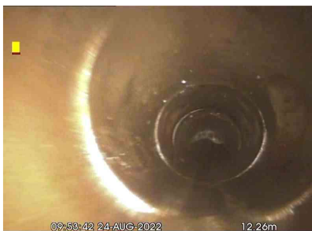
FMH4X_cc543651-f991-4fbf-80b3-b1434c4b92b7_20220826_141926_019.jpg, 00:00:41, 12.26 m Junction at 3 o'clock, 100mm dia
