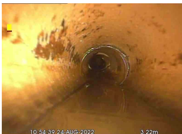
MH5aX_41d07ac9-d9c4-4869-9bb7-9788e3fc5b47_20220826_142943_326.jpg, 00:00:16, 3.22 m Water level, 10% of the vertical dimension
