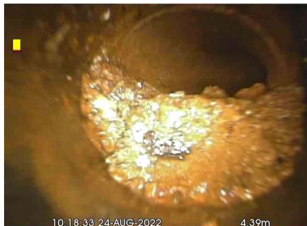
AX_2e6446a5-cc8a-4fc6-97dd-6214c854a780_20220831_090858_943.jpg, 00:00:22, 4.39 m Attached deposits, fouling from 4 o'clock to 8 o'clock, 60% cross-sectional area loss
