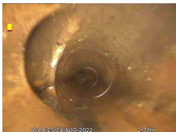
AX_714b0301-ffff-4b39-8712-293769aeea37_20220831_0900 26_932.jpg, 00:00:14, 2.77 m Junction at 9 o'clock, 100mm dia
