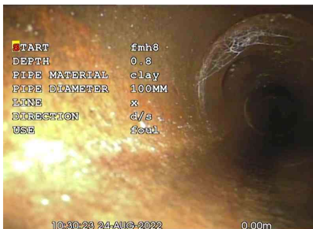
FMH8X_223f5c17-2ce0-4053-9505-8ae00a081fe1_20220831_142353_574.jpg, 00:00:00, 0.00 m Start node, manhole, reference: FMH8
