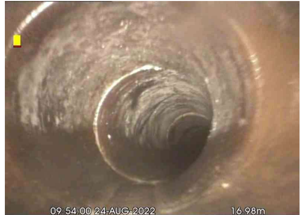
FMH4X_33add05e-5e43-4749-bb94-44b17bb806a5_20220826_142142_418.jpg, 00:00:59, 16.98 m Line deviates right
