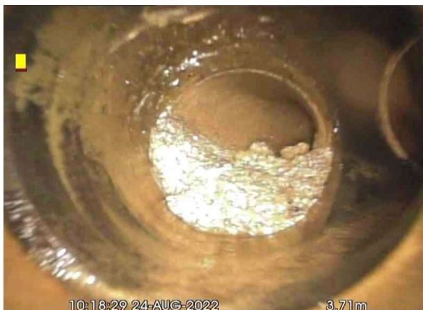
AX_2704cce3-6c8d-4109-9012-aa64dd096d45_20220831_090046_808.jpg, 00:00:17, 3.71 m Junction at 3 o'clock, 100mm dia
