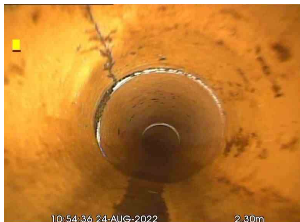
MH5aX_8c73f97d-d529-49aa-b717-17aa70eb161c_20220826_142925_823.jpg, 00:00:12, 2.30 m Roots, fine at joint
