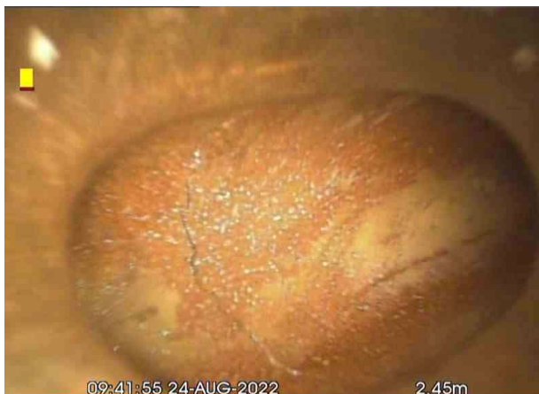
FMH3X_21f5451c-be09-4a81-8812-a3f63d96a9f9_20220826_121033_094.jpg, 00:00:13, 2.45 m Line deviates right, Junction on to secondary main
