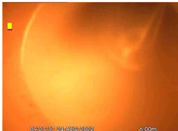
AX_667d7ead-8e06-44bf-b4ac-76761eb8275f_20220826_104 501_722.jpg, 00:00:24, 6.00 m Line deviates up
