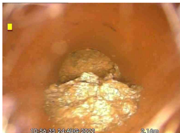
CX_d38bf258-8cdb-428f-bb34-b1031d1f510b_20220830_120 557_855.jpg, 00:00:10, 2.16 m Settled deposits, hard or compacted, 90% cross-sectional area loss
