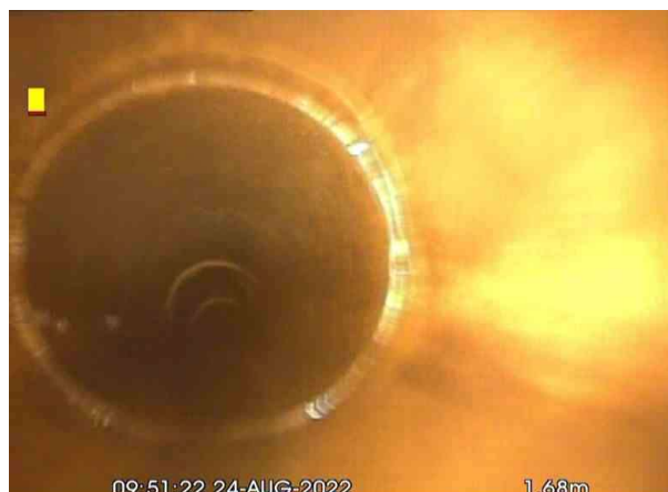
FMH5X_368cfac7-d831-4cc0-90fe-85dd2ab0d1e2_20220826_124459_799.jpg, 00:00:11, 1.68 m Crack, circumferential at joint from 9 o'clock to 3 o'clock
