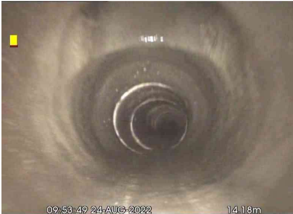
FMH4X_6c26063d-3ac3-4a37-9971-b9b53f614eaf_20220826_142014_936.jpg, 00:00:48, 14.18 m Junction at 12 o'clock, 100mm dia
