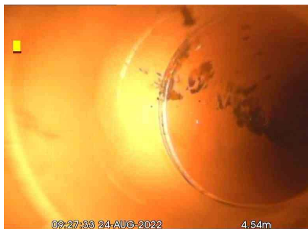
AX_b66f36bc-0cfb-48b7-8262-cbbbac2262e2_20220826_104 243_891.jpg, 00:00:20, 4.54 m Line deviates right
