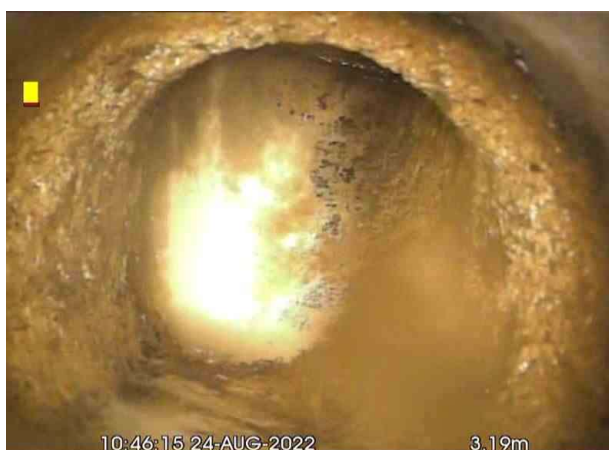
BX_6c7af187-6507-419c-a1c8-22f003c56d64_20220830_123935_478.jpg, 00:00:16, 3.19 m Line deviates up
