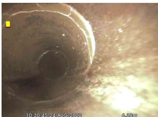
FMH8X_47d7b19c-1066-4d7b-844c-254ab95222e2_20220831_145604_091.jpg, 00:00:26, 6.33 m Crack, circumferential at joint from 9 o'clock to 4 o'clock
