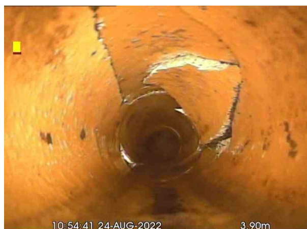
MH5aX_5680e134-a02a-4e76-8f4a-ba76ad208263_20220826_143019_247.jpg, 00:00:17, 3.90 m Broken pipe from 10 o'clock to 4 o'clock
