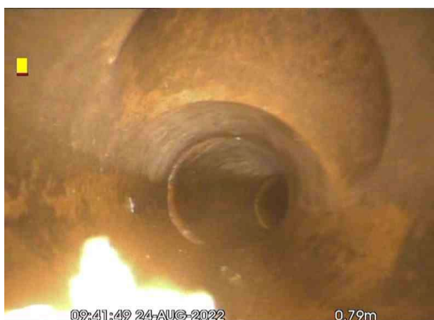
FMH3X_37bd1521-fe68-4c26-ab9b-9476fb9badb1_20220826_120953_355.jpg, 00:00:07, 0.79 m Junction at 12 o'clock, 100mm dia
