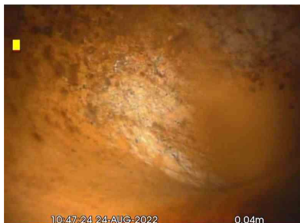
DX_1b5567a1-2938-4ff0-afdd-c0d29b063a3b_20220831_084 006_335.jpg, 00:00:06, 0.04 m Line deviates up
