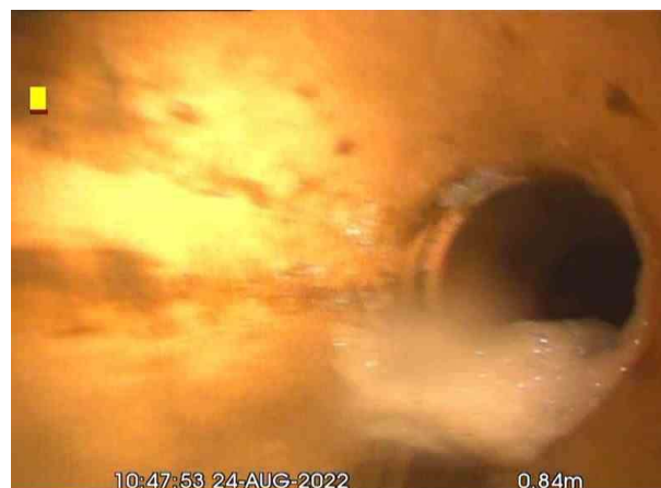
FMH6X_29790e47-512a-4eda-b7a0-491f57237c0f_20220831_084246_157.jpg, 00:00:07, 0.84 m Line deviates right
