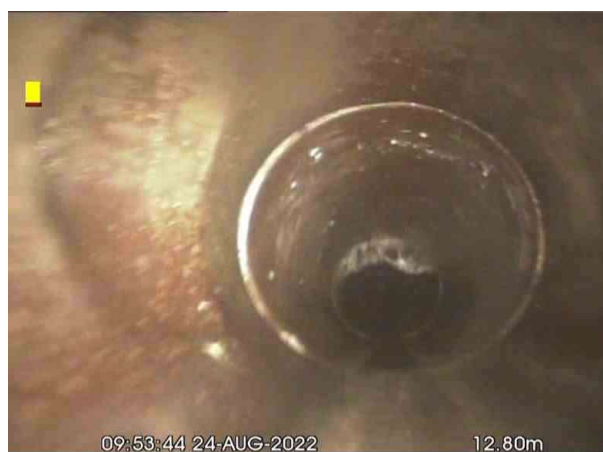
FMH4X_e97644c5-db3c-48b9-aa78-c2b2a3132fb6_20220826_141954_683.jpg, 00:00:43, 12.80 m Junction at 9 o'clock, 100mm dia
