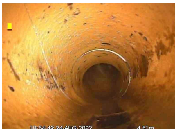
MH5aX_f90a0f58-68e0-404b-a191-e9604e2f41a0_20220826_143227_066.jpg, 00:00:23, 4.51 m Cracks, spiral from 7 o'clock to 11 o'clock
