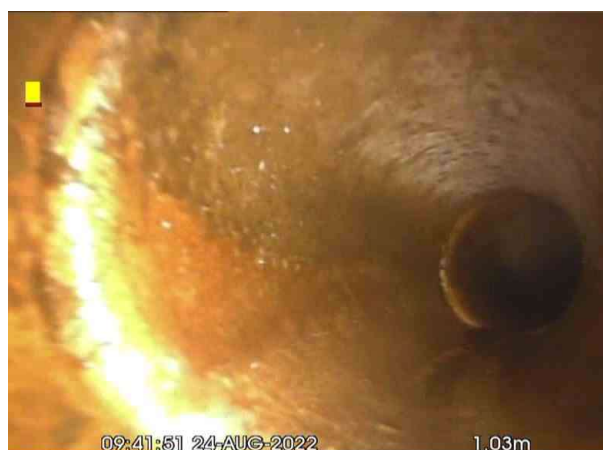
FMH3X_4356a4ec-7d7c-44e7-b8e5-65add26ca597_20220826_121004_884.jpg, 00:00:09, 1.03 m Line deviates right
