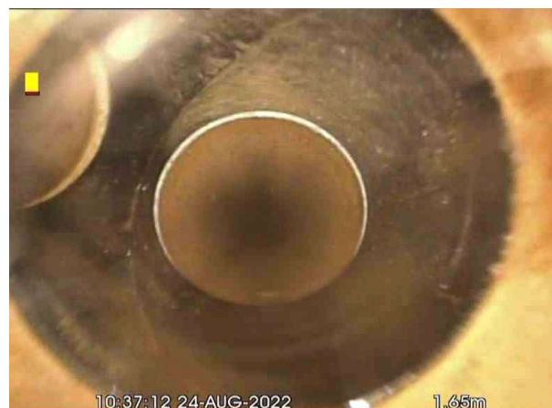
BX_624ca70e-b251-4dea-83eb-c4dae055e49c_20220901_09 0019_433.jpg, 00:00:11, 1.65 m Junction at 10 o'clock, 100mm dia
