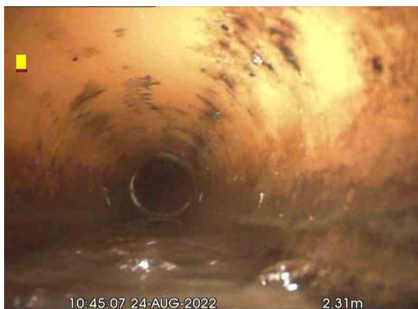
AX_1c5577ba-f5bc-414e-9412-db59d4d92daa_20220830_12 2110_240.jpg, 00:00:14, 2.31 m Water level, 5% of the vertical dimension
