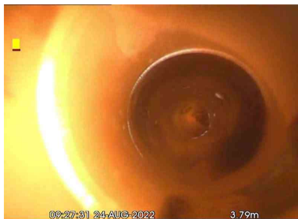
AX_a152e9e8-e048-4573-a99a-20447036e6e5_20220826_10 4047_112.jpg, 00:00:18, 3.79 m Junction at 1 o'clock, 100mm dia
