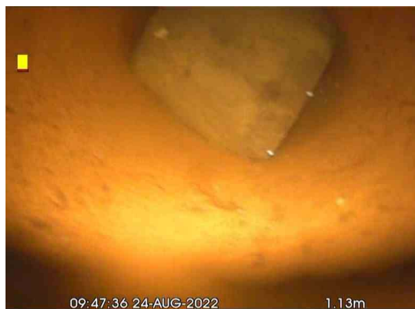
AX_c502f8ce-308e-4eca-8ddb-2a150e208aa8_20220826_123 949_533.jpg, 00:00:16, 1.13 m Finish node, other special chamber, reference: A, End of Survey / Suspected Capped off
