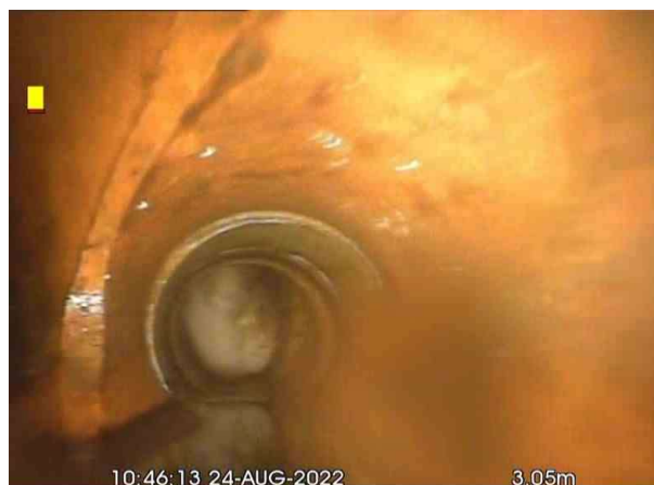
BX_60c548bf-789f-483f-9b0d-0cbf1cc3838a_20220830_123537_374.jpg, 00:00:15, 3.05 m Junction at 9 o'clock, 100mm dia
