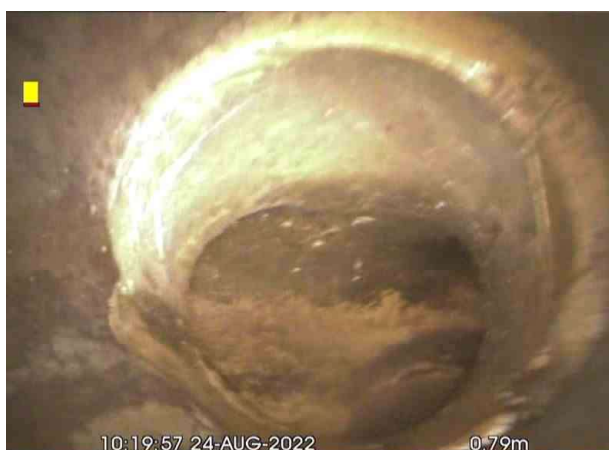
FMH7X_f9cedc1c-d439-4f12-8ebf-7563401176b6_20220831_111527_376.jpg, 00:00:10, 0.79 m Line deviates right
