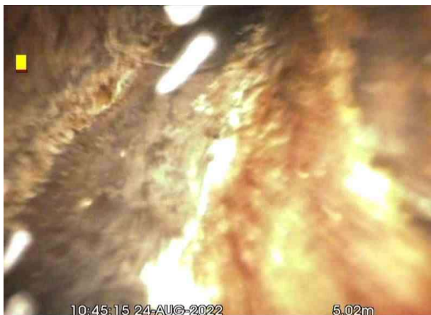
AX_39e1e0c9-407b-4d76-b147-21194ecba6c6_20220830_122210_028.jpg, 00:00:23, 5.02 m Line deviates up
