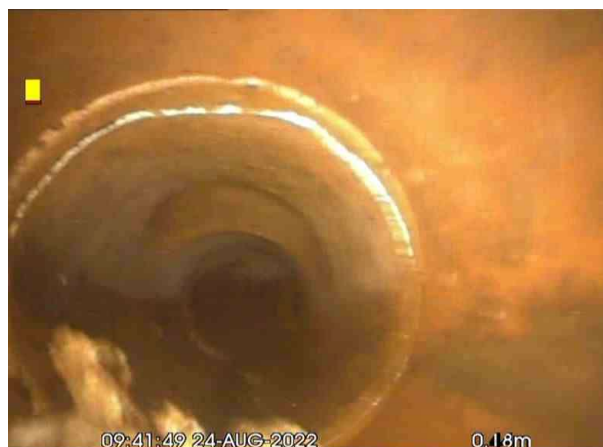
FMH3X_3c744aaa-f794-492d-8fe9-5964c65f8630_20220826_120929_486.jpg, 00:00:07, 0.18 m Fracture, circumferential at joint from 9 o'clock to 3 o'clock
