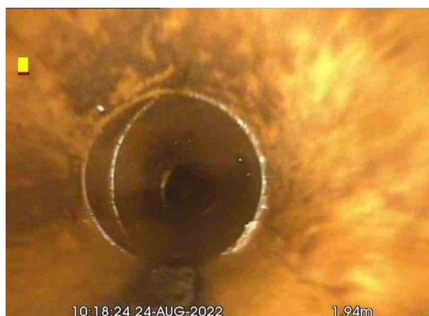
AX_0fa8d69e-d375-409f-ba34-bd15a1b1a549_20220831_085 940_765.jpg, 00:00:13, 1.94 m Fracture, circumferential at joint from 7 o'clock to 11 o'clock
